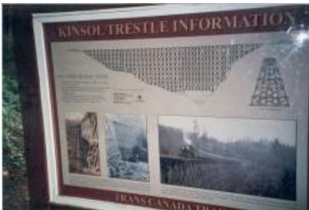
Kinsol Trestle on TransCanada Trail Nov. 04/05 (Cowichan River) Vancouver Island (815 ft. long 125 ft. above the Koksish River) Largest wooden trestle in the British Commonwealth. The construction started in 1911. All the timbers were cut and left at the site. Construction was halted due to 1 st World War. After the War the timbers left on site had deteriorated and had to be replaced. The trestle was completed in 1920. It was last used in 1979.
